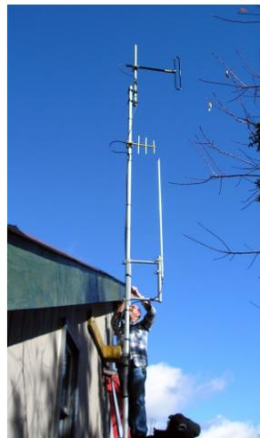
The pipe holds the new Telewave repeater antenna (top), the UHF link Yagi, and an APRS antenna, bottom
